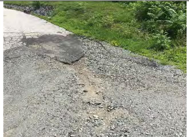
**Photo 1:** Sediment runoff directly into the Poultney River channel.
